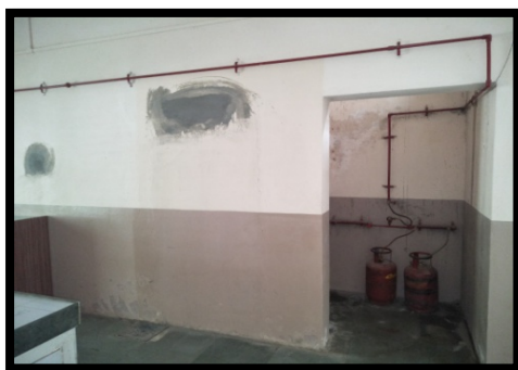
Fig. 7.5 Gas connection pipe line in lab and Transformer protective shield
